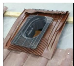
Cut the underlay diagonally as a cross shape as shown above, then pin the underlay back to surrounding battens and rafters. Position the vent into the cut hole.
