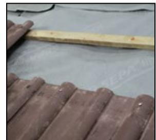
Position the Tile vent where required and ensure the vent is directly in line with the tile below. (Do not at this stage lay tile to either side). Use the vent to draw the template to mark the hole.
