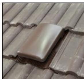
Once Tile Vent is dressed to the tile, clip the cap onto the base securely. Carry on tiling as normal
