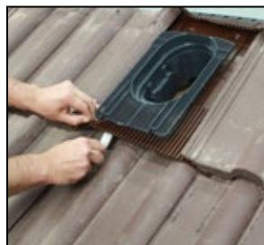
All Tile Vent has to be mechanically fixed down in line with BS 5534 as shown in the photos above. Lay tiles to both sides of base once nailed. Remove protective tape and dress skirt to the profile of the tile
