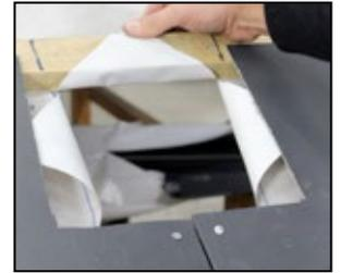
Mark the position for the Slate Vent by drawing a box with a cross as shown above. Place the adjacent slate and mark the required size to cut the slates.
