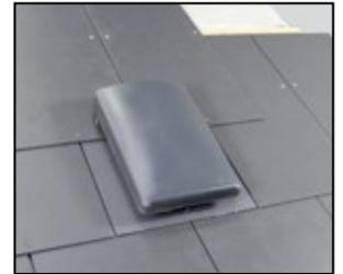
Slide the vent - spigot first - into the opening. Using the centring line on the vent, align with the joint line of the two slates directly below. Fix vent by nailing through centre nail holes. Place the adjacent slates around the Slate Vent accordingly.
